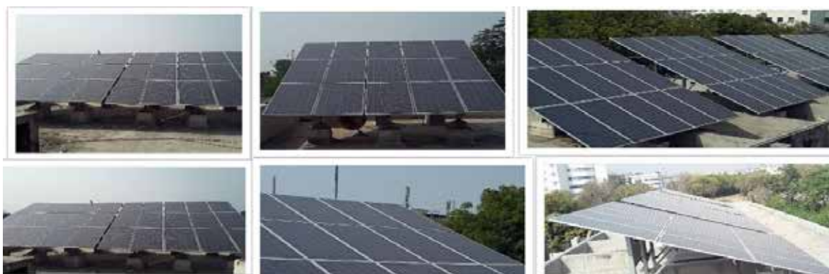
Figure 33 A Green Initiative by NHB Installation of Roof Top Solar Panel at NHB Building
